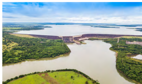
Brazil São Simão Hydropower Plant
