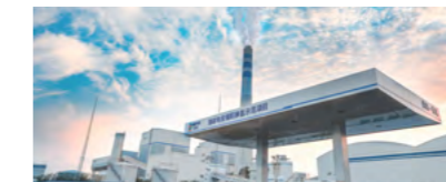
Chaoyang HCNG Demonstration Project
